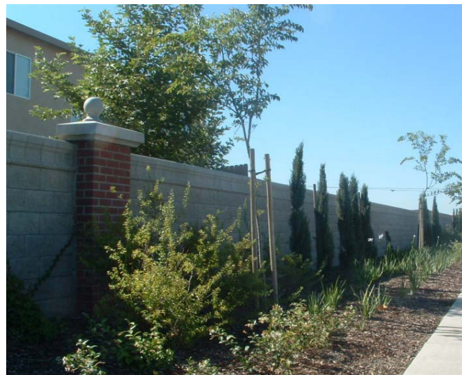
Rear yard and interior side yard walls shall be no higher than 6 feet.
