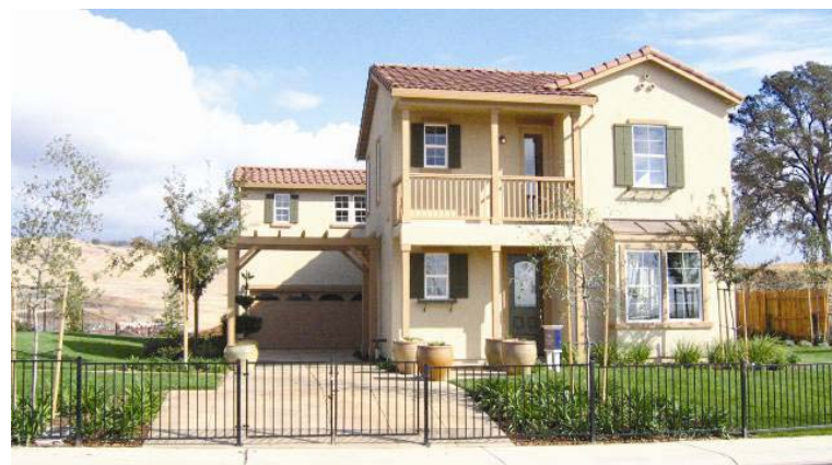
Locating the garage behind the front facade of the house is encouraged.
