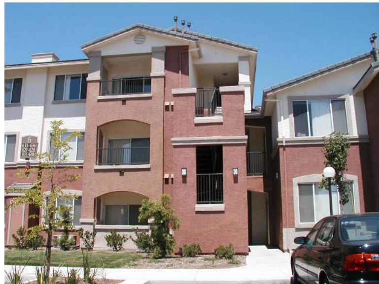
Projecting balconies and changes in color and material add interest and break up large facades.
