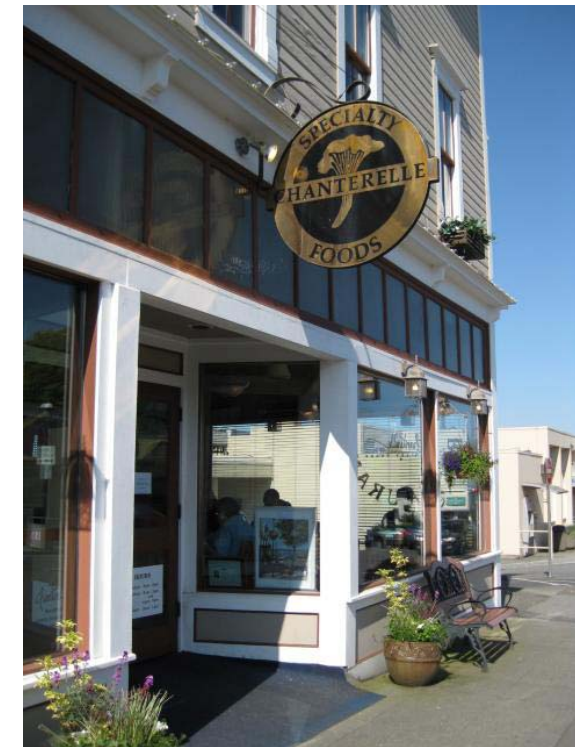
Traditional storefront features include bulkheads, display windows and recessed entries.
