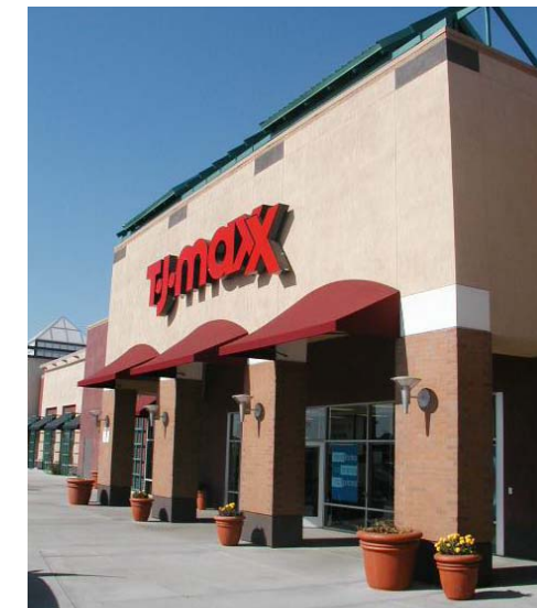
Base of building incorporates change in color and material.
