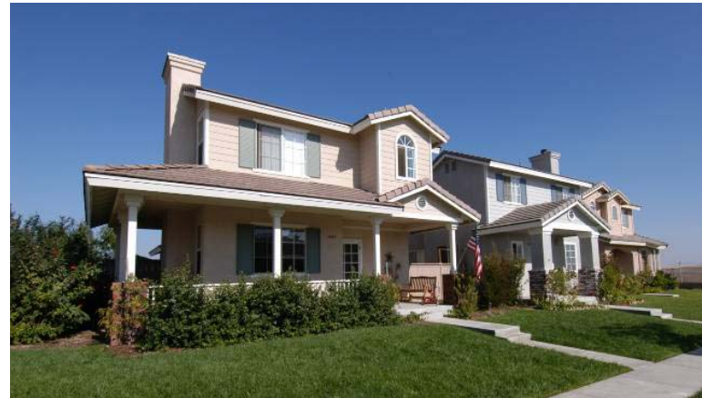
These homes feature porches, a single-story element that provides a transition in two-story massing.
