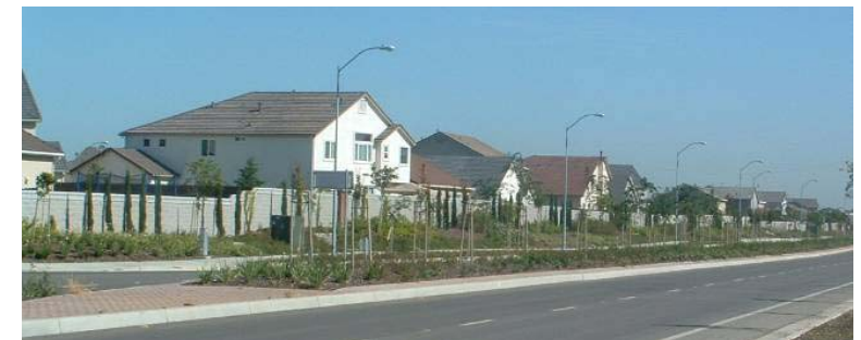
Perimeter walls adjacent to major arterials must be of masonry construction and should have a minimum 10-foot landscaped setback.
