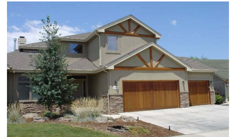
Three-car garages should be designed so that the third garage is architecturally separated.
