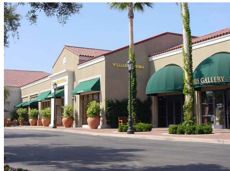
Gabled and hipped roofs.
