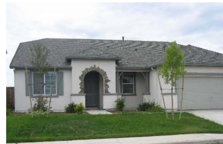
Entries should be the focal point through the use of porticos, pop-outs or other architectural features.
