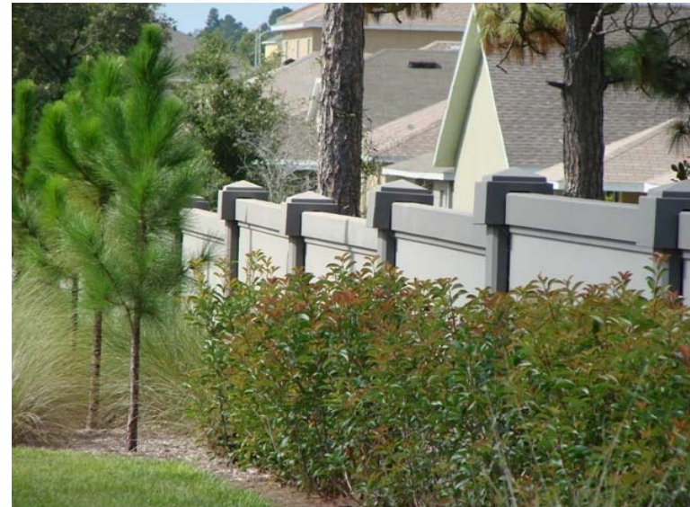
Perimeters walls should incorporate various textures, staggered setbacks, architectural elements, and variations in height in conjunction with landscaping to provide visual interest and to soften the walls' appearance.
