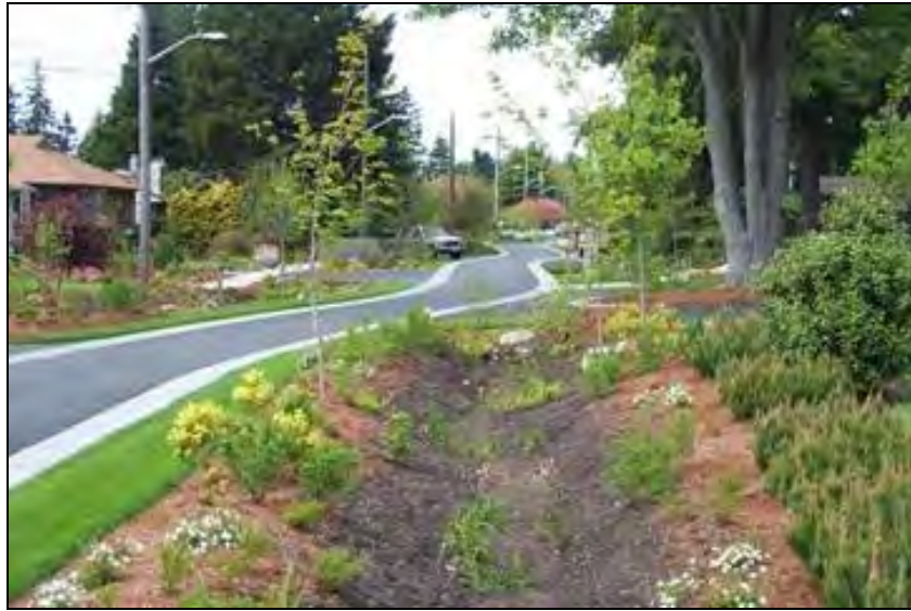
Figure PUBLIC-5 Roadside Drainage Swale
