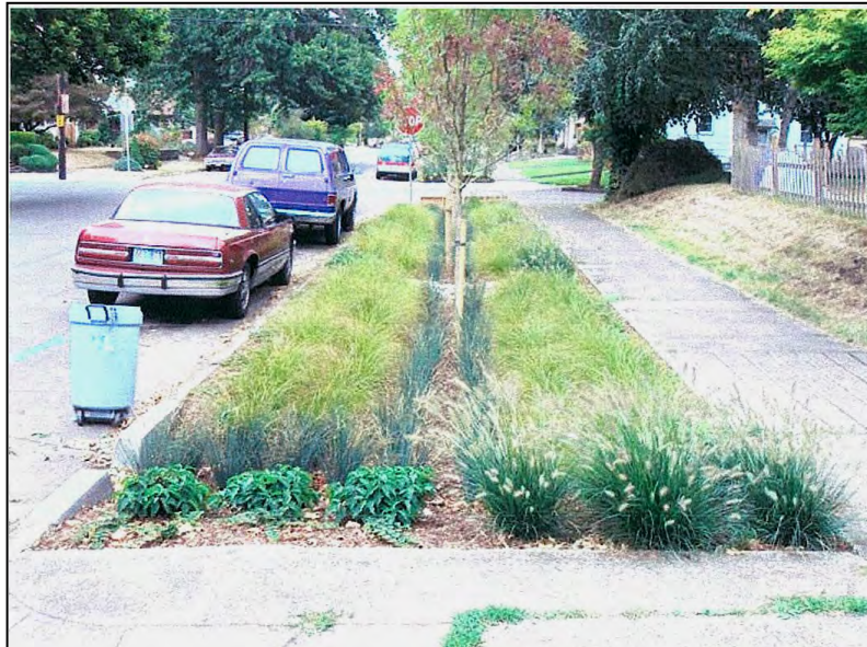
Figure PUBLIC-6 Planter Strip Stormwater Infiltration
