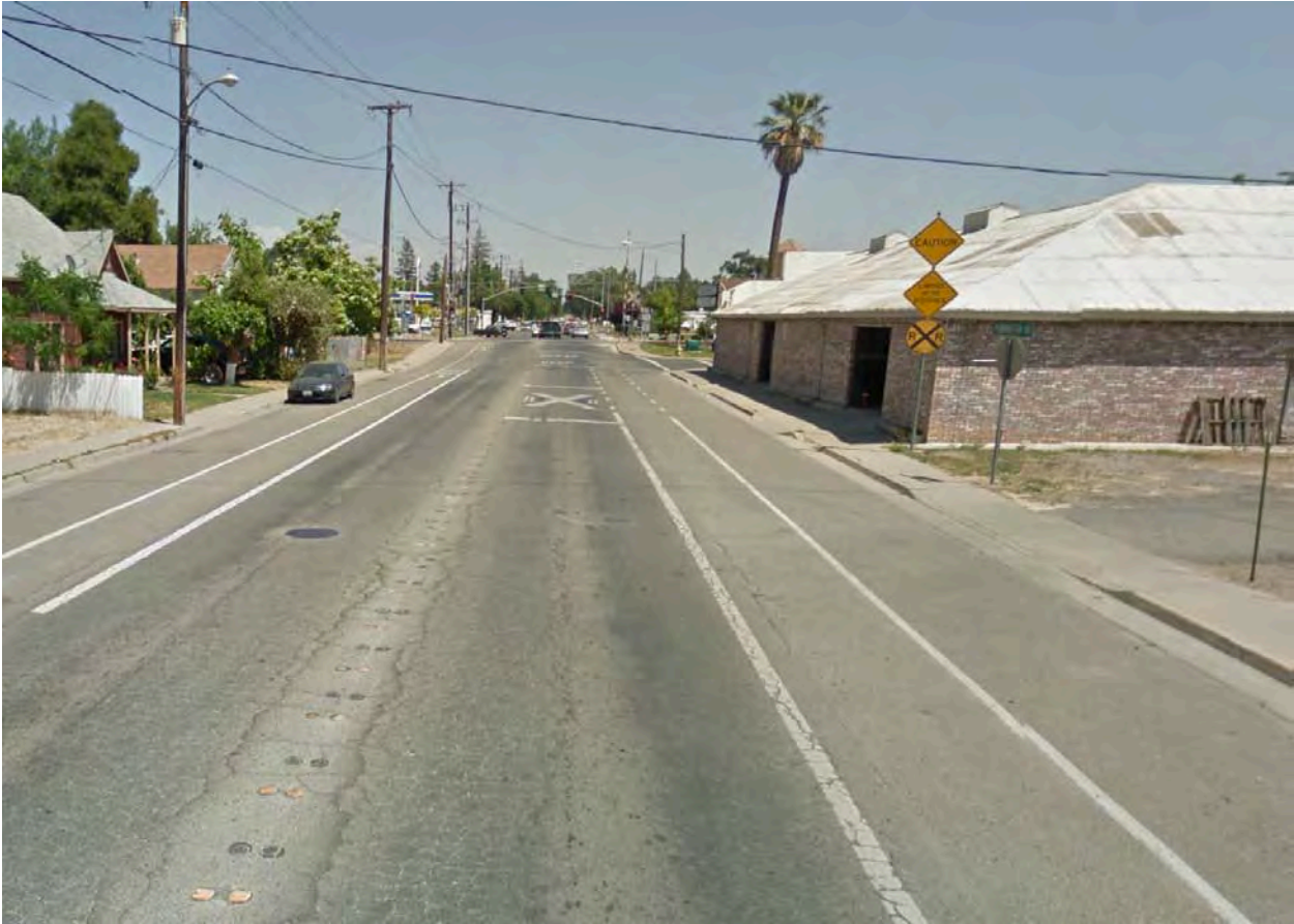
Figure 3 - Pennington Rd. looking east from N St.
