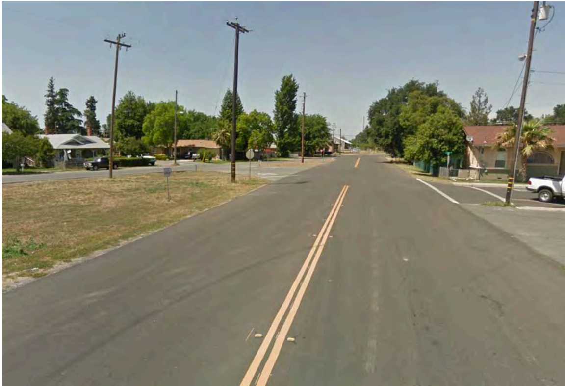
Figure 6 - California St. looking N/W at Gum St.
