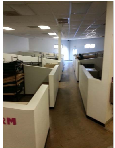
Figure 10. Housing Unit C/D interior partitions
