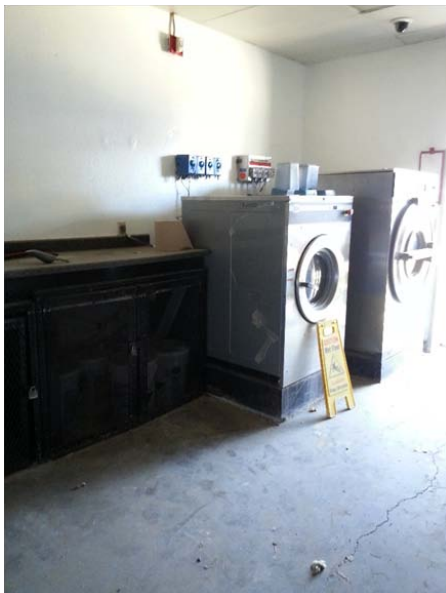
Figure 25. Laundry room interior
