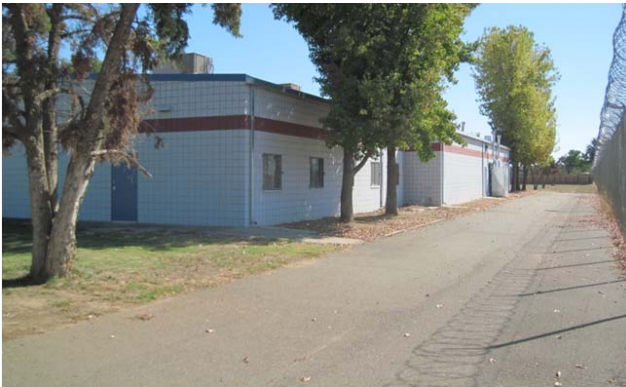
Figure 6. Asphalt paving on west side
