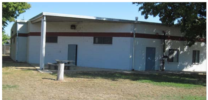
Figure 9. Housing Unit C/D west wall, northwest corner
