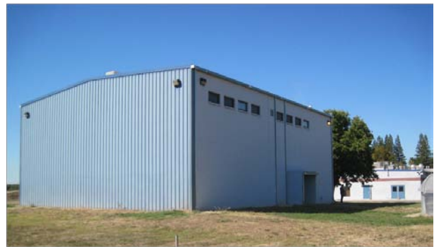
Figure 22. Gymnasium south and east walls
