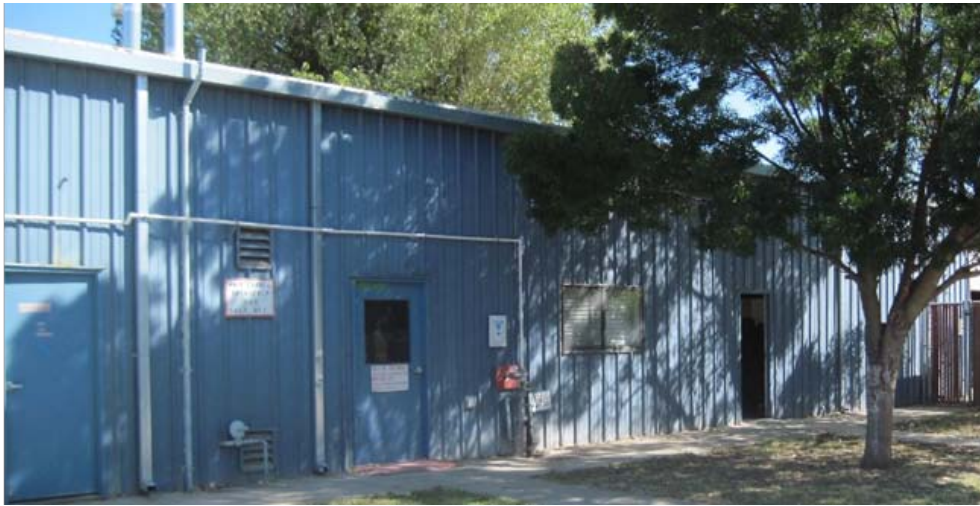
Figure 24. Maintenance / Laundry west wall
