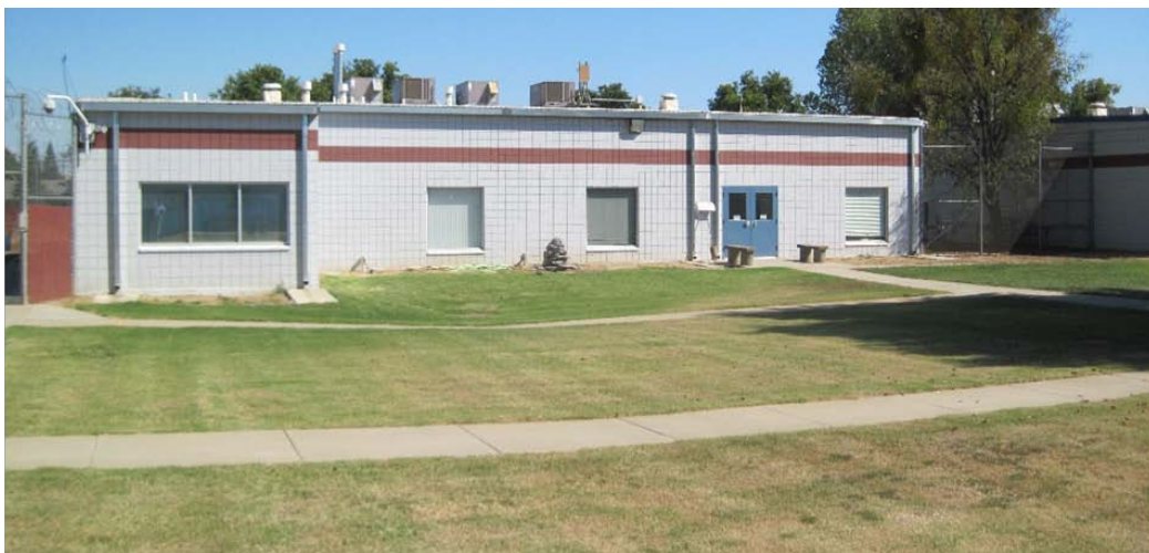
Figure 15. Administration west wall
