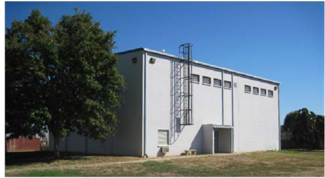
Figure 19. Gymnasium north and west walls
