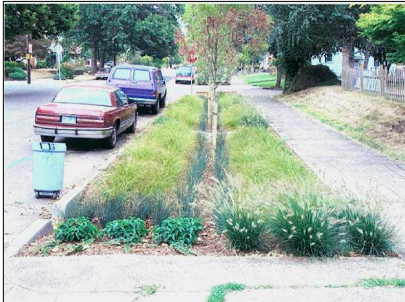
Figure PUBLIC-6 Planter Strip Stormwater Infiltration
