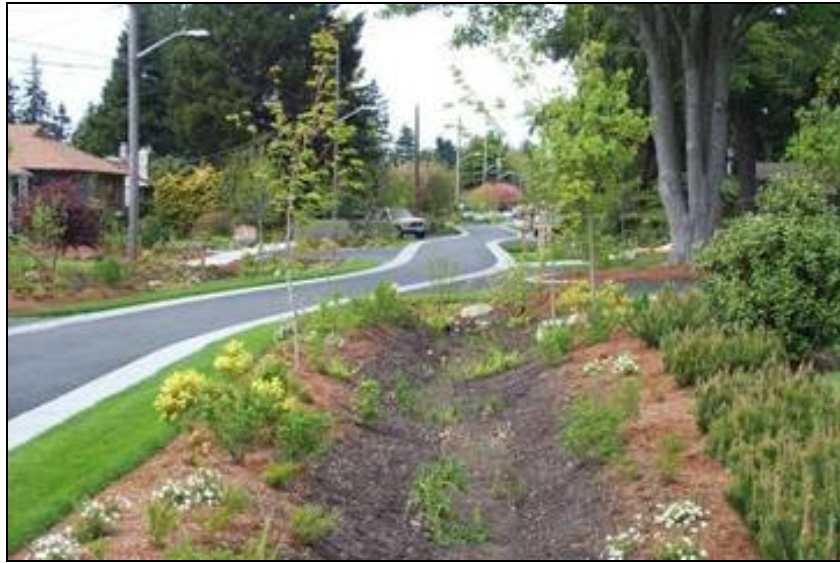
Figure PUBLIC-5 Roadside Drainage Swale
