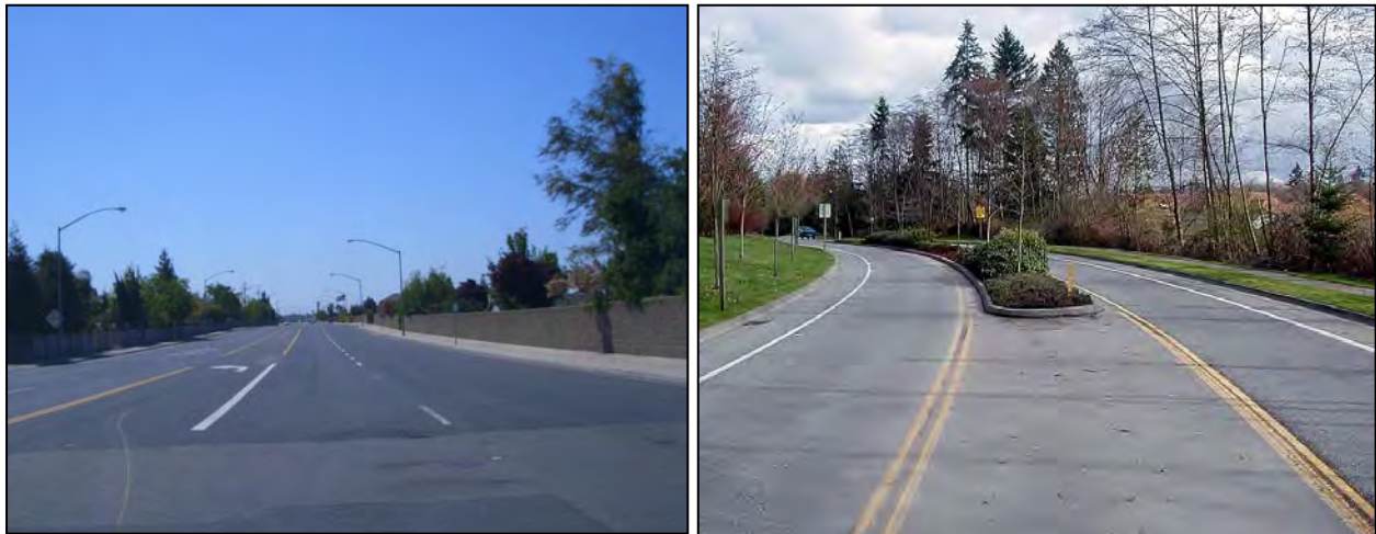
Figure DESIGN-7 Overly wide collector streets should be avoided (Left); Collector streets can function well with narrower travel lanes for vehicles (Right)
