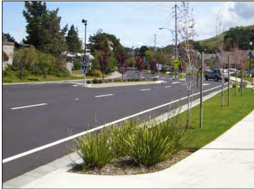
Figure DESIGN-8 Collector street with landscaped median and planting strip, street trees, and separated sidewalk
