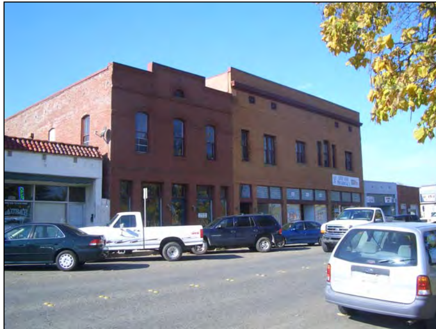
Figure DESIGN-24 Existing historical buildings should be preserved and adaptively reused
