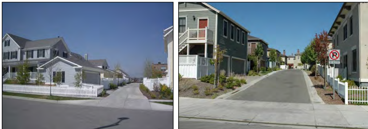
Figure DESIGN-3 Alleyways may be provided for garage access, second units, and services
