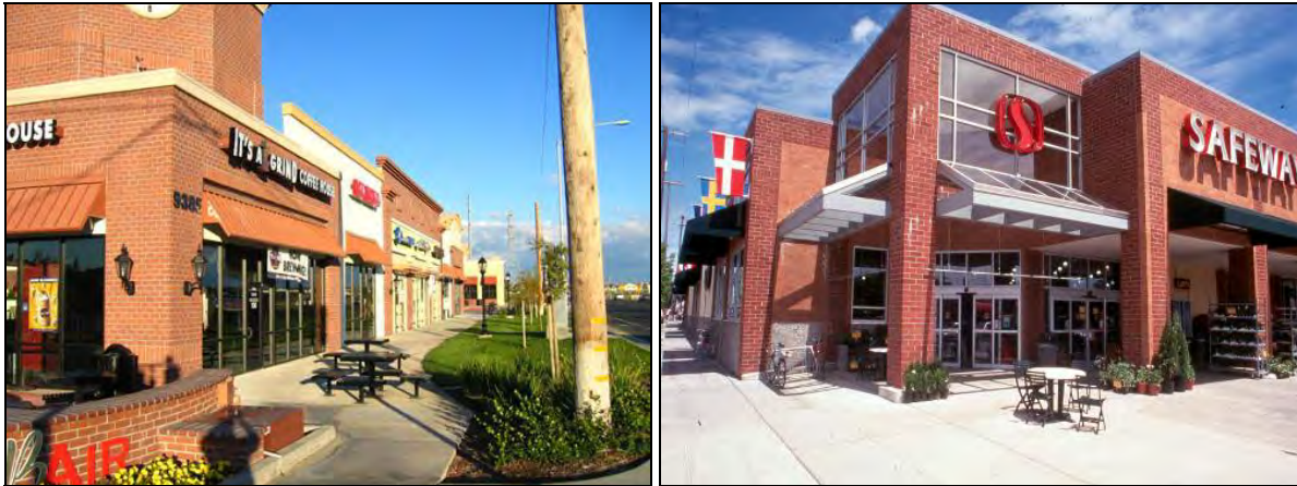
Figure DESIGN-28 Retail uses should face and open onto sidewalks and plazas
