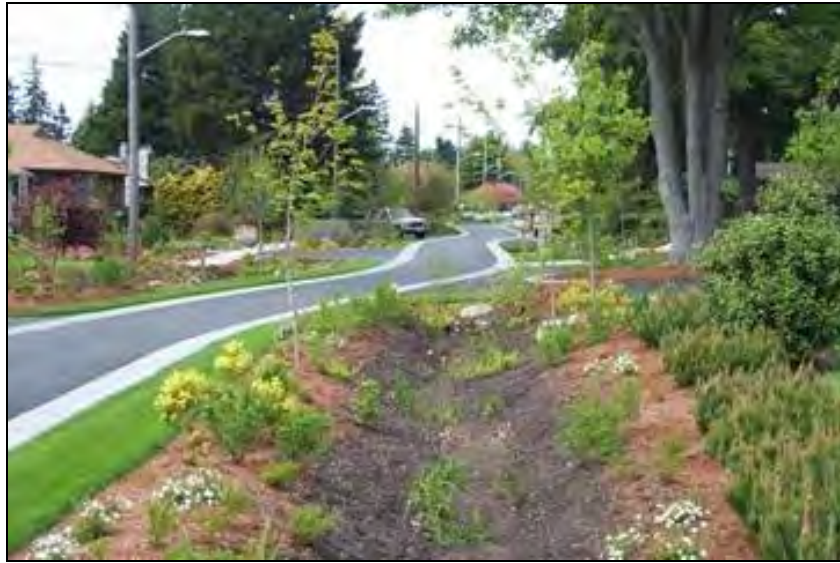
Figure PUBLIC-5 Roadside Drainage Swale
