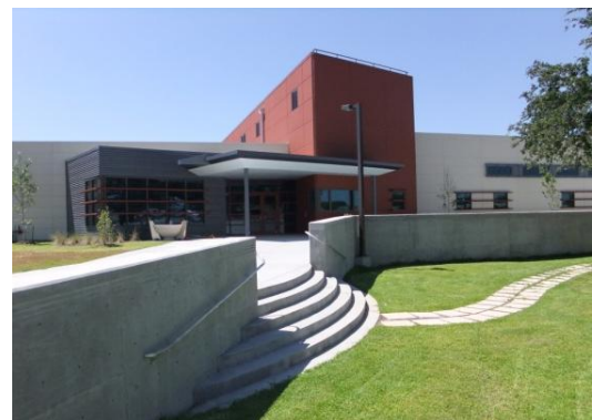
Photo 3 - Flood Protected Communication Center, New Orleans
