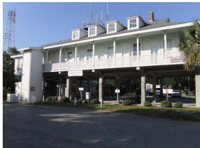
Photo 5 - Flood Protected Town Hall, Grand Isle, La.
