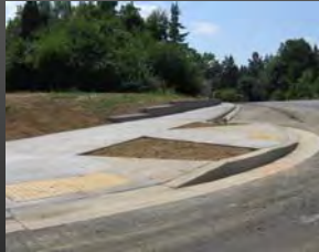
Depressed parking next to travel lanes.
