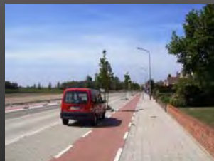
Distinguished paving on pedestrian and bike ways adjacent parking.
