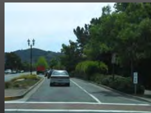
Separated sidewalk with landscaped parkway, paved crosswalk, median and dedicated bike lane.
