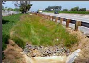
Engineered bioswale next to travel lanes separated with guard rails..
