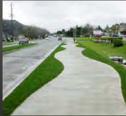
Grassy strip separating combined bike/pedestrian way with a grassy swale and drainage to the interior side.
