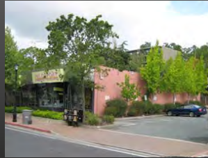
Parking at the side of the building.
