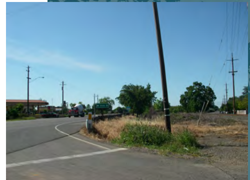
Existing crowning on the highway causes visual hazard.
