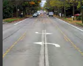
Dedicated bike lane with separated sidewalks and landscaping adjacent travel lane.
