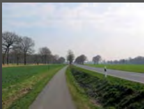
Stormwater drainage ditch along Highway with separates bike and pedestrian way.
