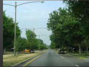
Dedicated landscaping along Highway with separated sidewalks; drainage within landscaped parkway.
