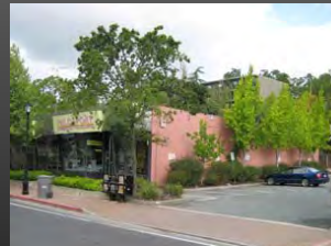
Parking at the side of the building.
