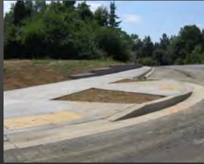
Depressed parking next to travel lanes.
